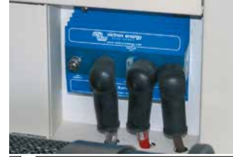
Engines battery charger
