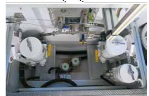
Fuel separator filters
