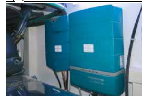
Service battery charger and inverter (optional)
